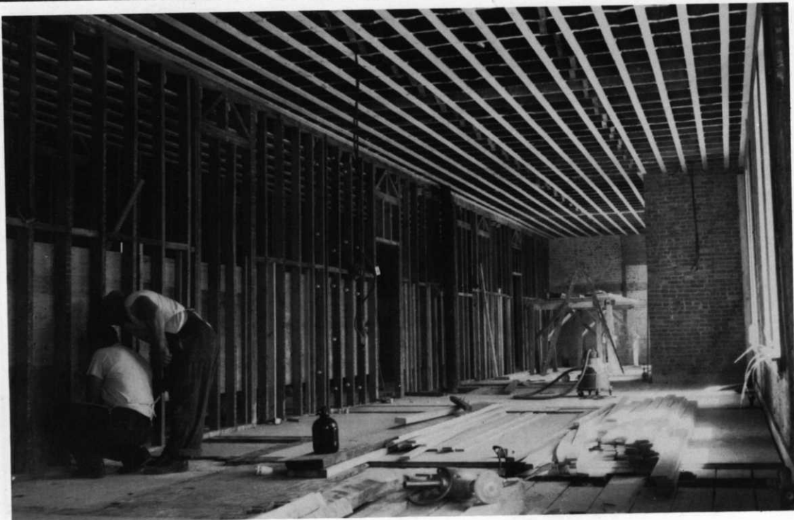
Remodeling the Dormitory
