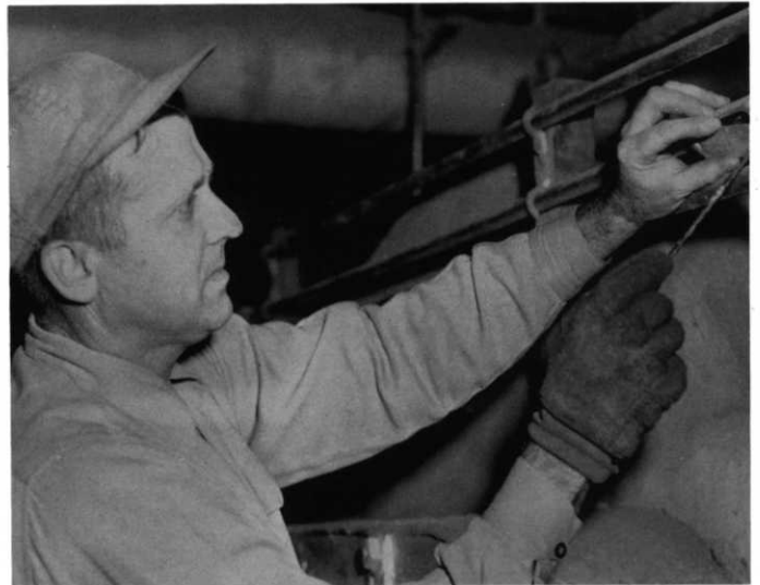
Brother Martin Bak, O.F.M. Boiler Room
