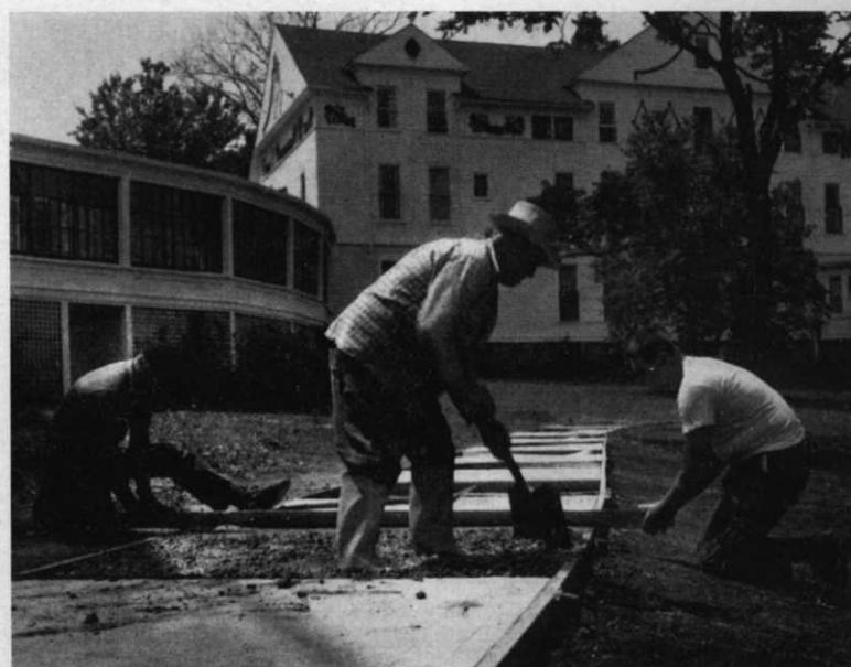
Brothers Timothy, Benedict and Simon laying the new sidewalk
